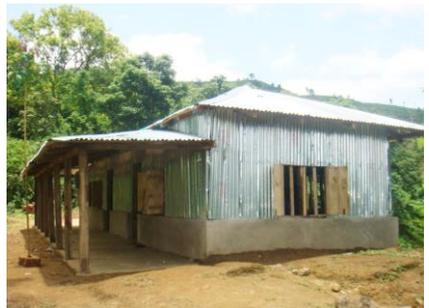
The school comprises two classrooms constructed from a locally cut timber frame and profiled steel sheets.
